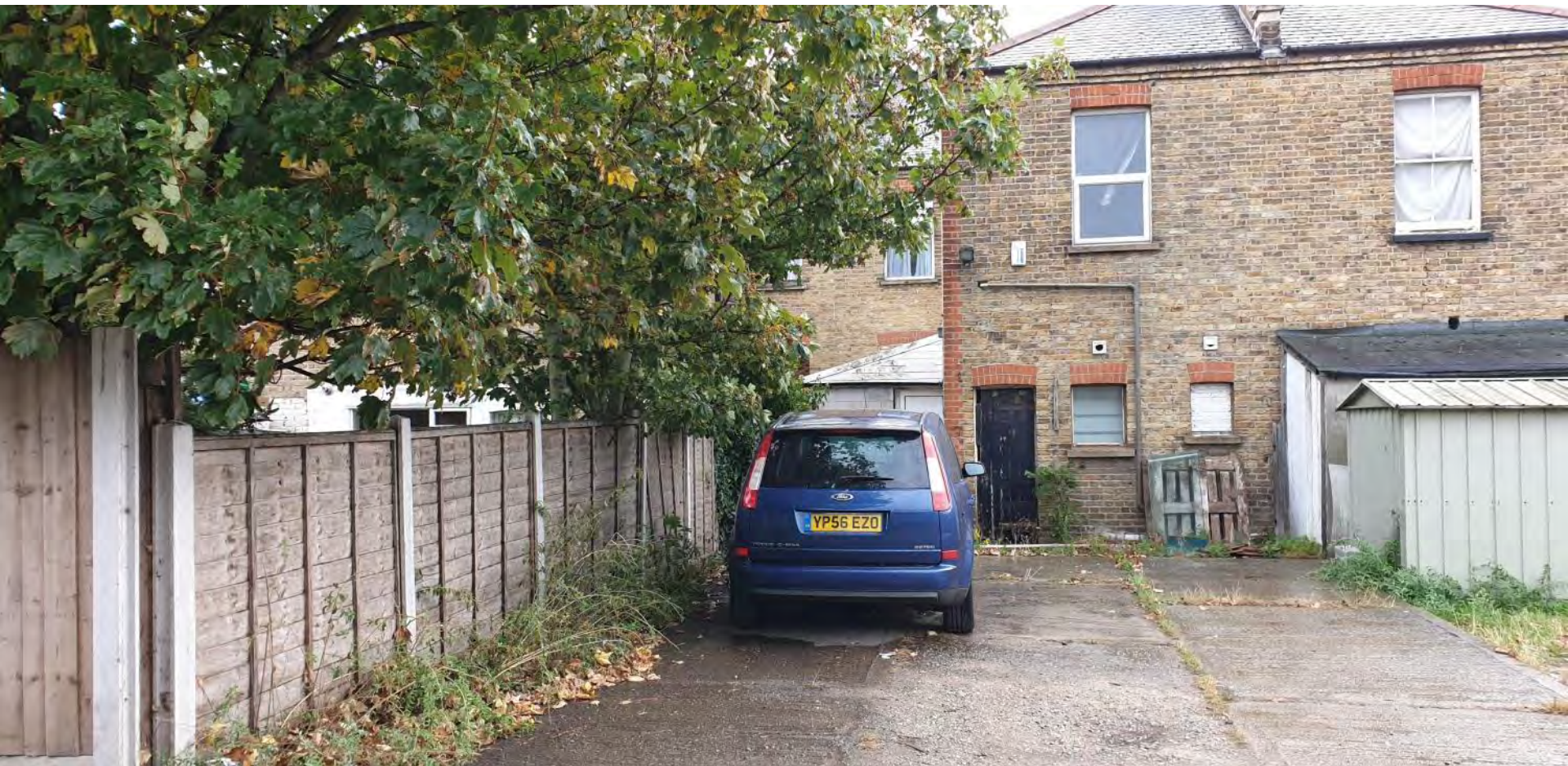
Rear of Southchurch Road units
