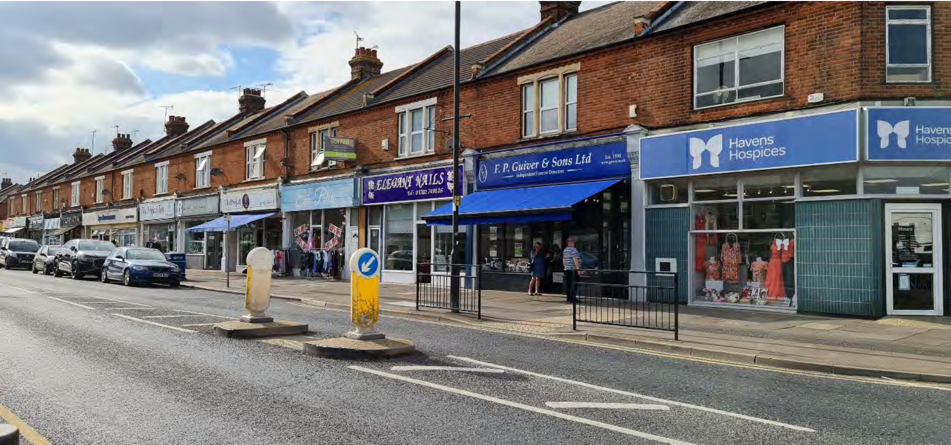
East end of Southchurch Road terrace
